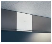
Presence detector, temperature sensor and  ${\rm CO_2}$ sensor are used for fully automatic control of lighting and ventilation
