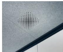
Fresh air is drawn into the room via an invisible sound absorber integrated in the acoustic ceiling
